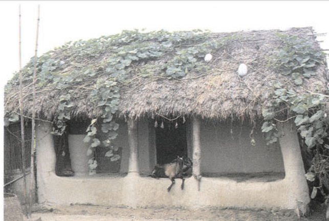
Fig. 17.6b Walls can be plastered to reduce harbourages.
