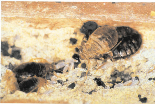
Fig. 11.8 Bedbug infestation. A prison cell had become infested, the bedbugs laying eggs in the mortar cracks on the wall. Nymphs and cast skins can also be seen.
