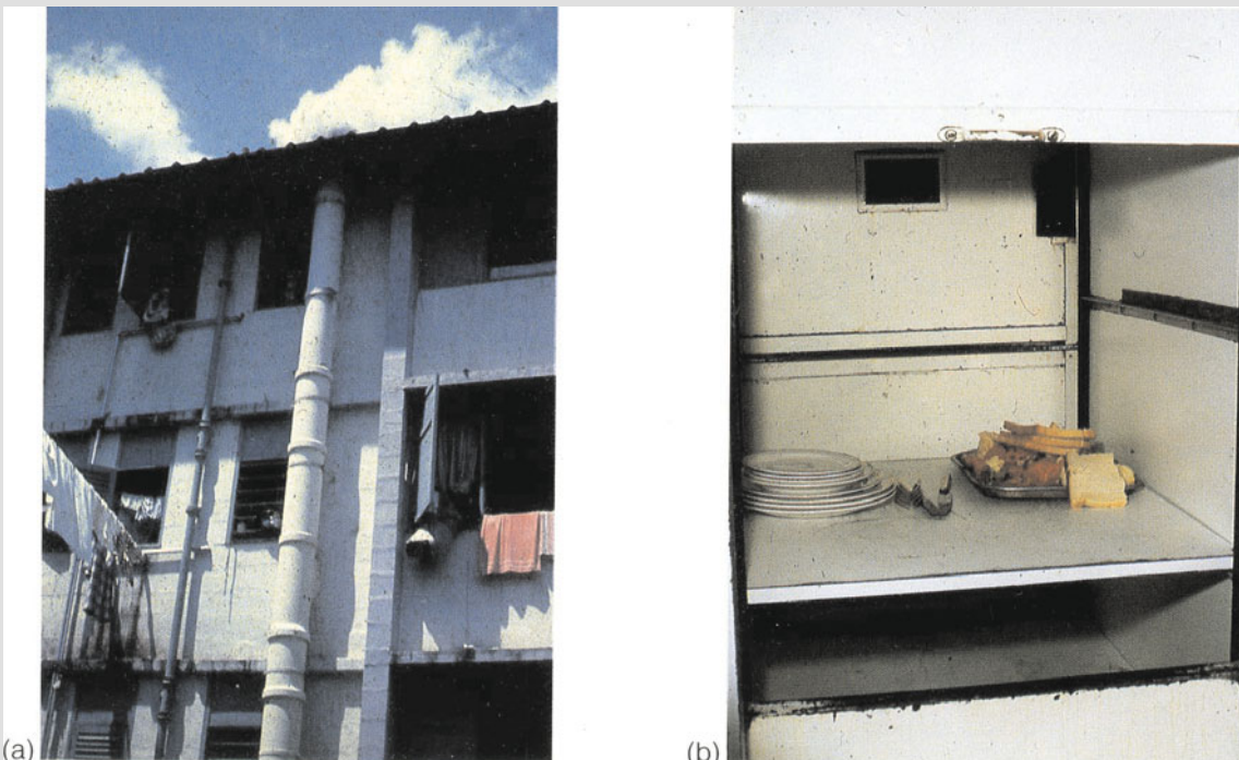
Fig. 17.20 Sites treated with insecticidal dust. (a) Ducting. (b) Lift-shafts.
