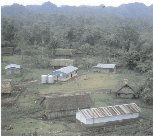
Fig. 17.6a Selection of building materials. Replacement of roofs with corrugated iron.
